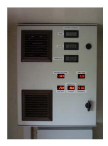
The controller for the wind turbine is sited in the drying room so that any waste heat during high winds can help to prevent freezing in winter.
