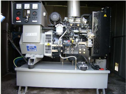
The generator is presently housed in a temporary shed while the permanent stone building is under construction. A simple lamp indicator system in the kitchen alerts the residents if the batteries are running too low and need charging from the generator.
