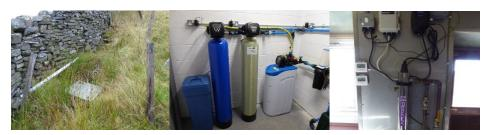
**Waste water** goes to a 3500 litre septic tank underground on the moor side of the building. The liquid run off from the tank is filtered naturally and the solids removed when the tank is emptied each year. We do not use any bleach or strong disinfectants which would prevent this process working properly.
